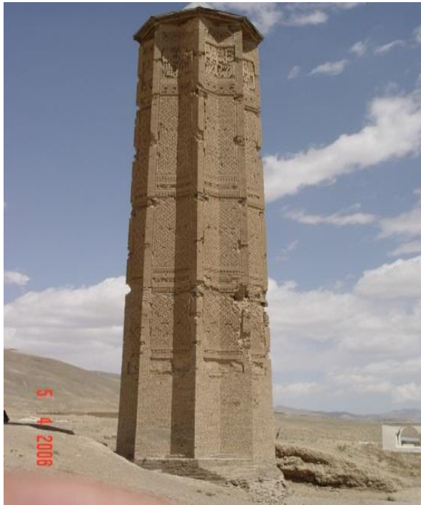
Figure 2. General view of the Minaret of Masoud III, copied from the book Review of Archaeological Excavations in Ghazni Province, 1396.
